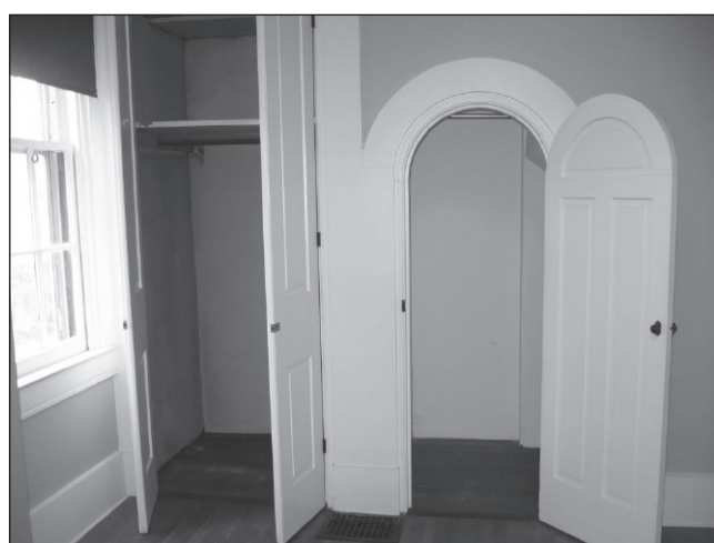
Since houses built at this time did not typically have closets, these were probably added during the 1920s. These closets are significant because the original large plank flooring dating from the house's construction still remain.
