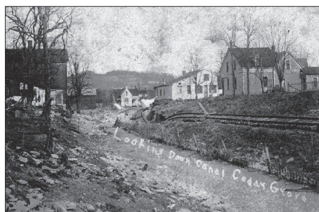
No historic renderings or drawings exist from the time the Whitewater Canal was in service through Rochester. This photo, taken after the 1913 Flood devastated the area, is the only one to date that explicitly identifies the canal in town. The railroad tracks seen to the right were laid on the old towpath of the canal. Image from the Shirley Seufert collection, FCPLD.
