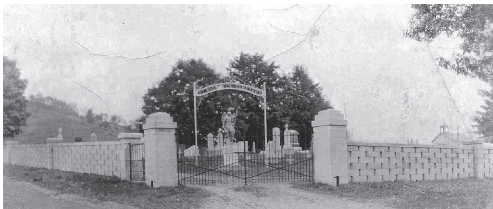
The Riedman Brothers concrete block wall surrounding St. Michael's Cemetery in Brookville. Courtesy Greg Pflum, FCPLD digital collection.
